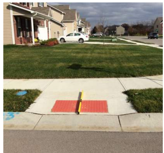
Running slope measurement is taken parallel to the direction of travel on a ramp.
