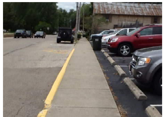
Use of parking blocks help prevent obstruction of sidewalk by overhanging vehicles.
