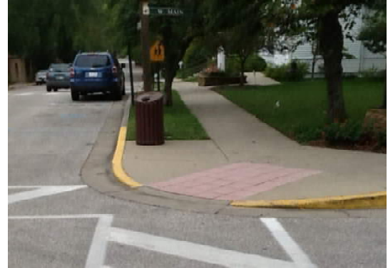
Room appears to be available for turning space/landing at top of ramp. Adequate space for bottom turning space at diagonal ramp may not wholly fit within cross walk.
