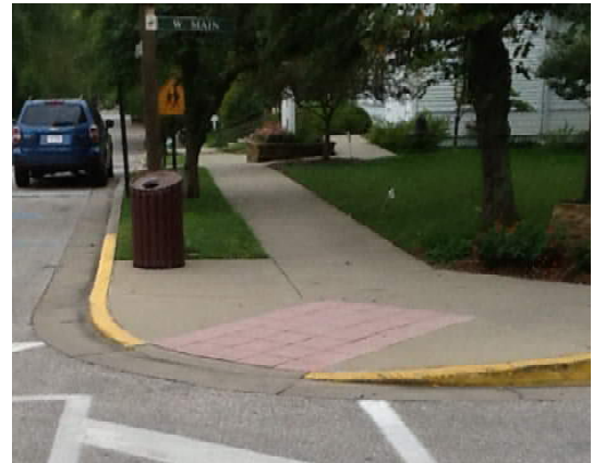
The pedestrian circulation area around both sides of this ramp necessitate use of a flare.
