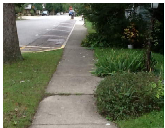
Vegetation overhanging from adjacent properties can obstruct required clear width.
