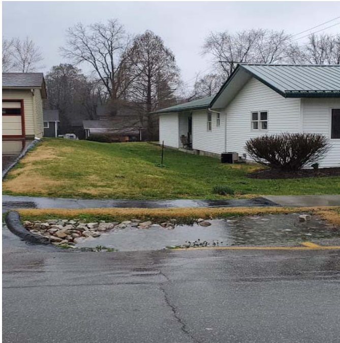
Looking at South Roadside of Main Street from Johnson Street
