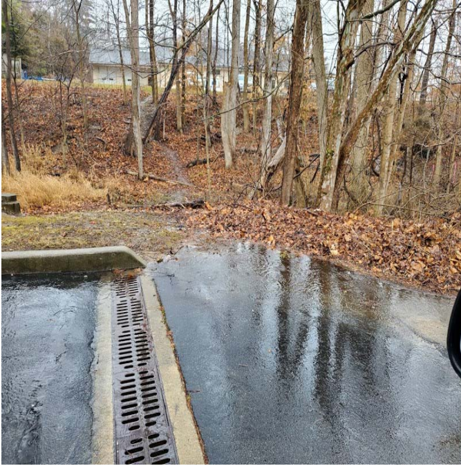
Looking at Conveyance Channel from East end of Gound Street
