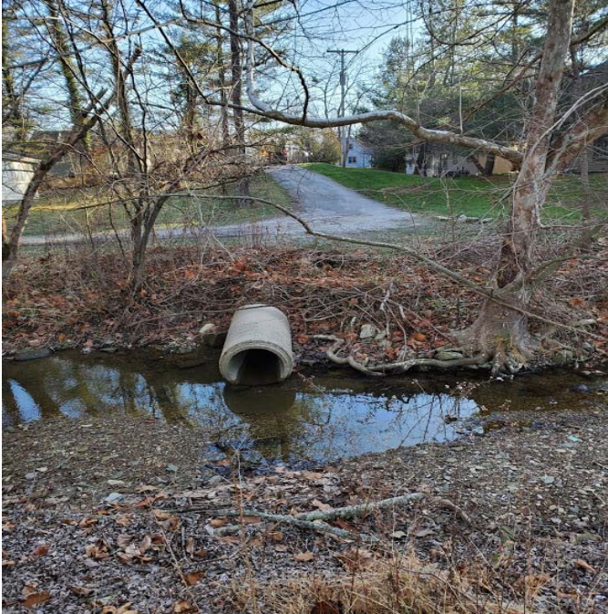
Looking East at Outfall into Jackson Branch at Gould Street
